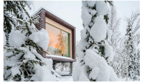
Nordic installations (heavy snow loads and up to -15°C)
