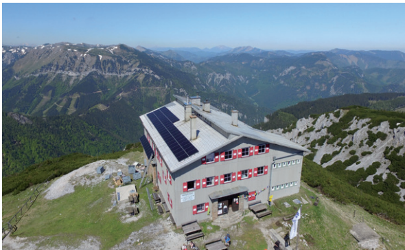
Mountain installations (strong wind pressure)
