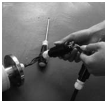
③ Fastening the cable cover.
